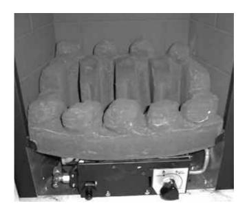
Position the front row of four loose coals along behind the first row of coals, ensuring that the flame paths as indicated are not interupted.
