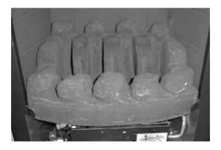
Position the front row of four loose coals along behind the first row of coals, ensuring that the flame paths as indicated are not interupted.
