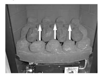
c) Fit the remaining three coals onto the ribs in the fuelbed as shown below, ensuring that the rear flame paths as indicated are not interupted See Fig. 14 below.
